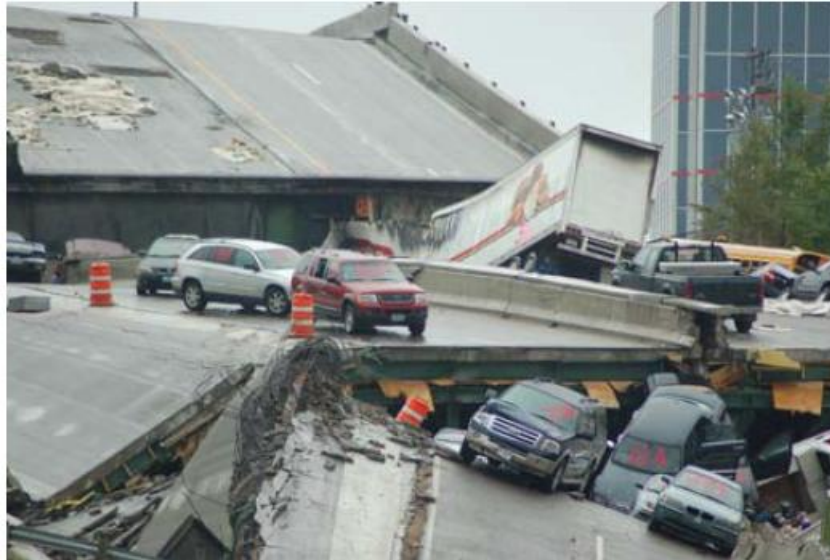
Figure 1.4: Bridge collapse in Minneapolis, 2007.
