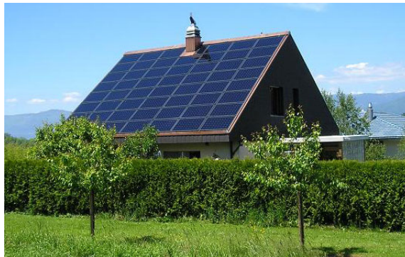
Figure 2.27: Installing solar panels on the roof of a house.
