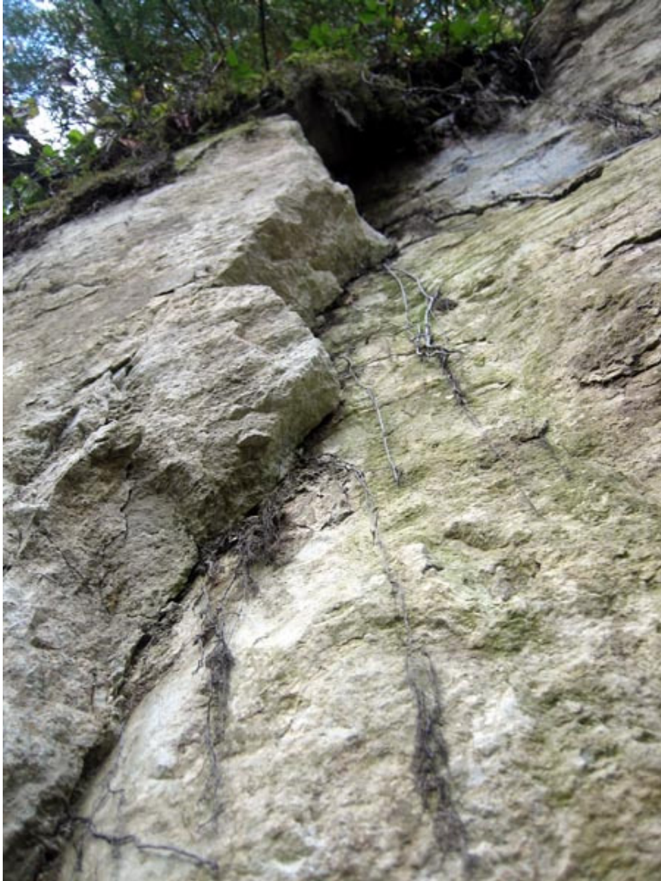
Figure 2.4. Photo of fractured bedrock along the logging road's cut-bank shown in Figure 2.2.
