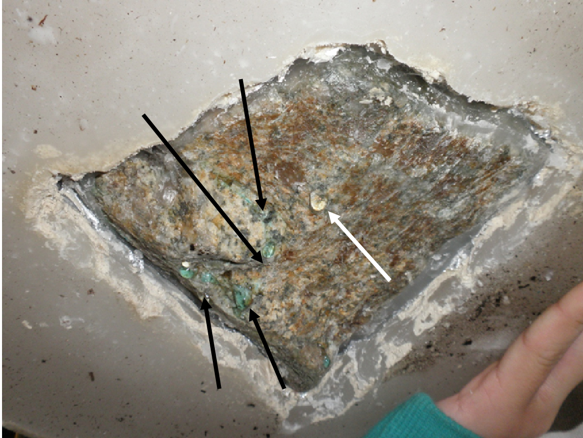
Figure 3.12. Photo of rock core T1. This figure shows preferential flow through fractures. Blue dye was introduced a week after the start of the falling head infiltration test. The clear water droplet shows that water is moving through the rock at different rates. Black arrows show locations of blue water drops and the white arrow shows the location of a clear water drop.
