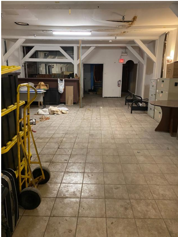
Figure 6.2: The restaurant storage space under the Silver Avalon Hotel.
