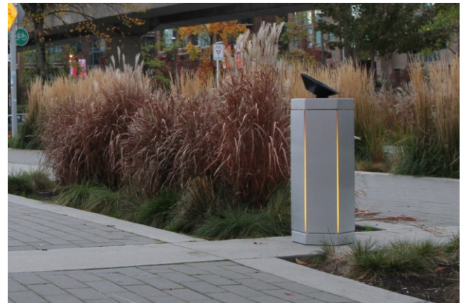
Figure 1. One of the three data posts during the installation.
