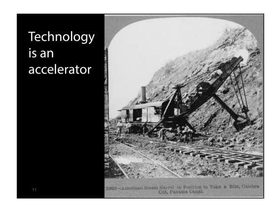
But when it came to building the Panama Canal a few years later, human effort was insufficient – and the harnessing of steam power in a new way, with the steam shovel, was the technology that accelerated canal building.
