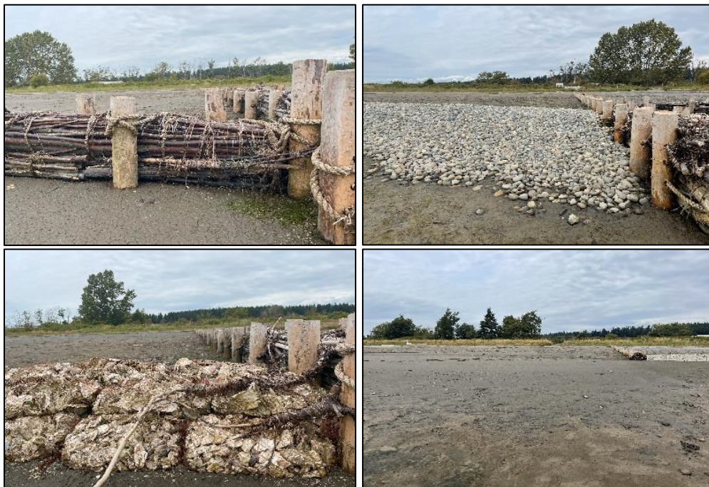
Figure 6: Image showing the four edge treatments at the S1 LDPP study site in Boundary Bay, British Columbia. Clockwise from the top left: brushwood dam, gravel berm, sand berm, oyster bag berm.
