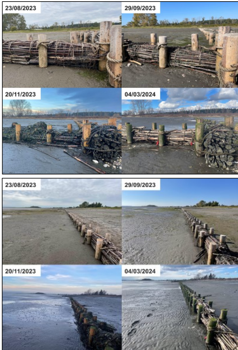
Figure 17: Photo monitoring of the brushwood dam treatment between August 23 rd , 2023 and March 4 th , 2024 at the S1 LDPP site in Boundary Bay, British Columbia. The March 4 th , 2024 image shows a repaired brushwood bundle.
