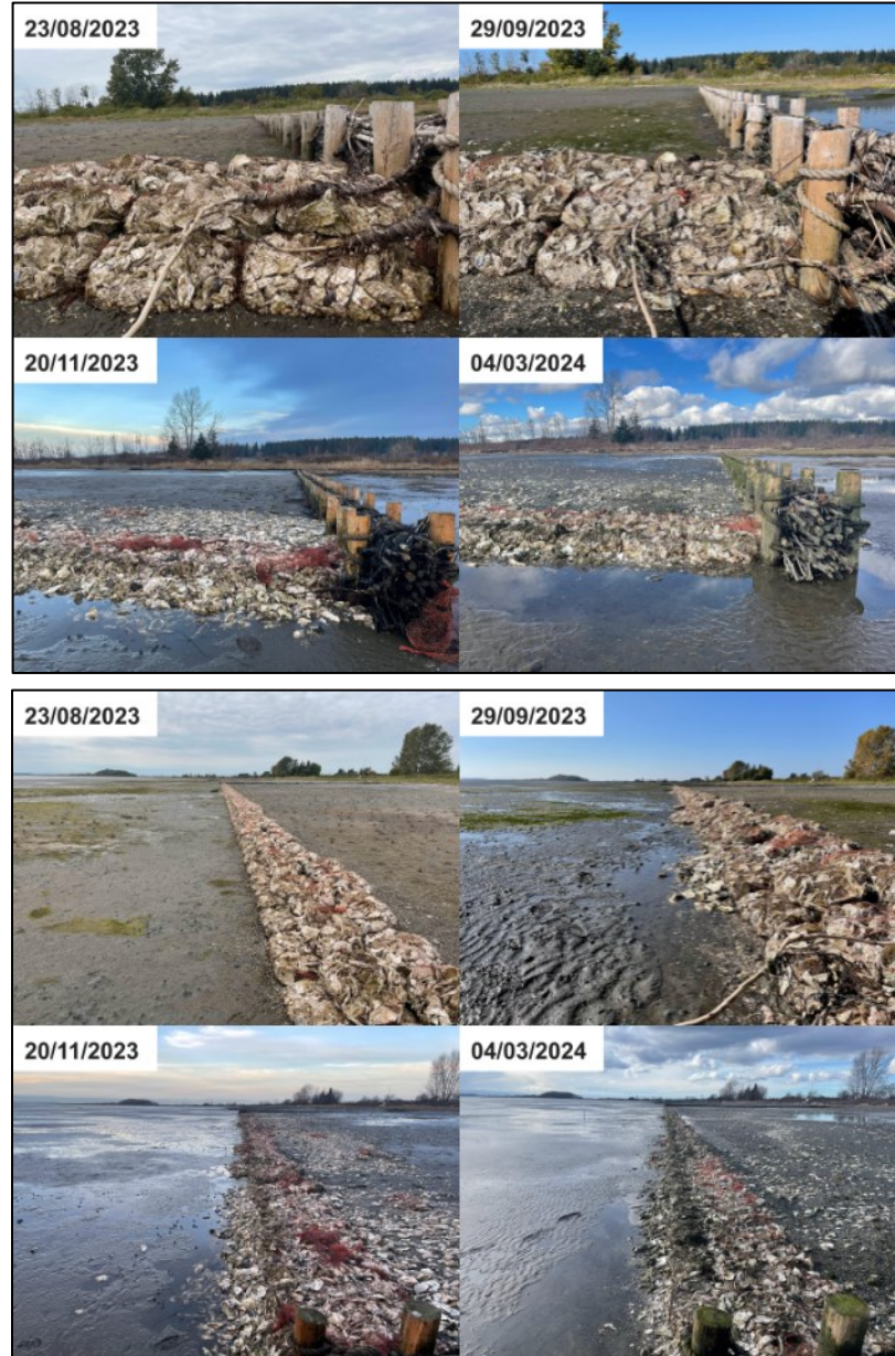
Figure 18: Photo monitoring of the oyster-shell bag berm treatment between August 23 rd , 2023 and March 4 th , 2024 at the S1 LDPP site in Boundary Bay, British Columbia.
