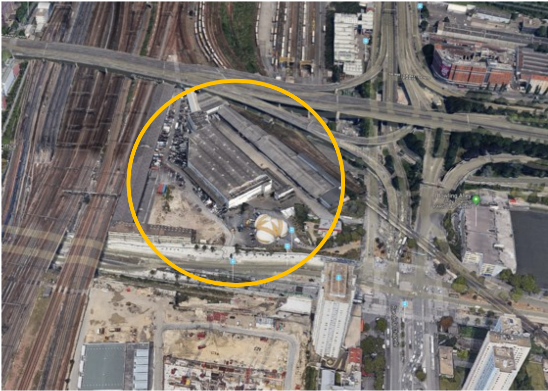
Figure 1.7 Satellite view: The CPA in Porte de la Chapelle, located between the boulevard Ney, the boulevard périphérique, and the train tracks in an abandoned hangar belonging to the national railway. Source: Google Earth.
