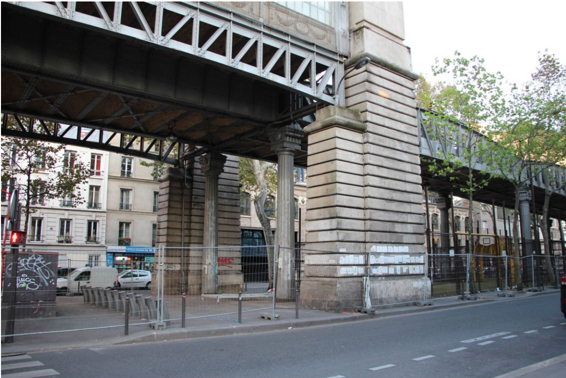
Figure 4.1 Fences installed under the aerial metro between the Stalingrad and Jaurès metro stations in the 10 th arrondissement of Paris to prevent migrants’ encampments, November 2017. Photo: Melora Koepke
