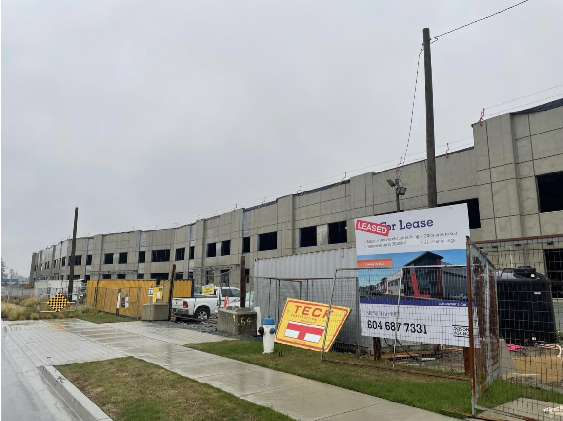
Figure 3-1. Warehouse development in Abbotsford
