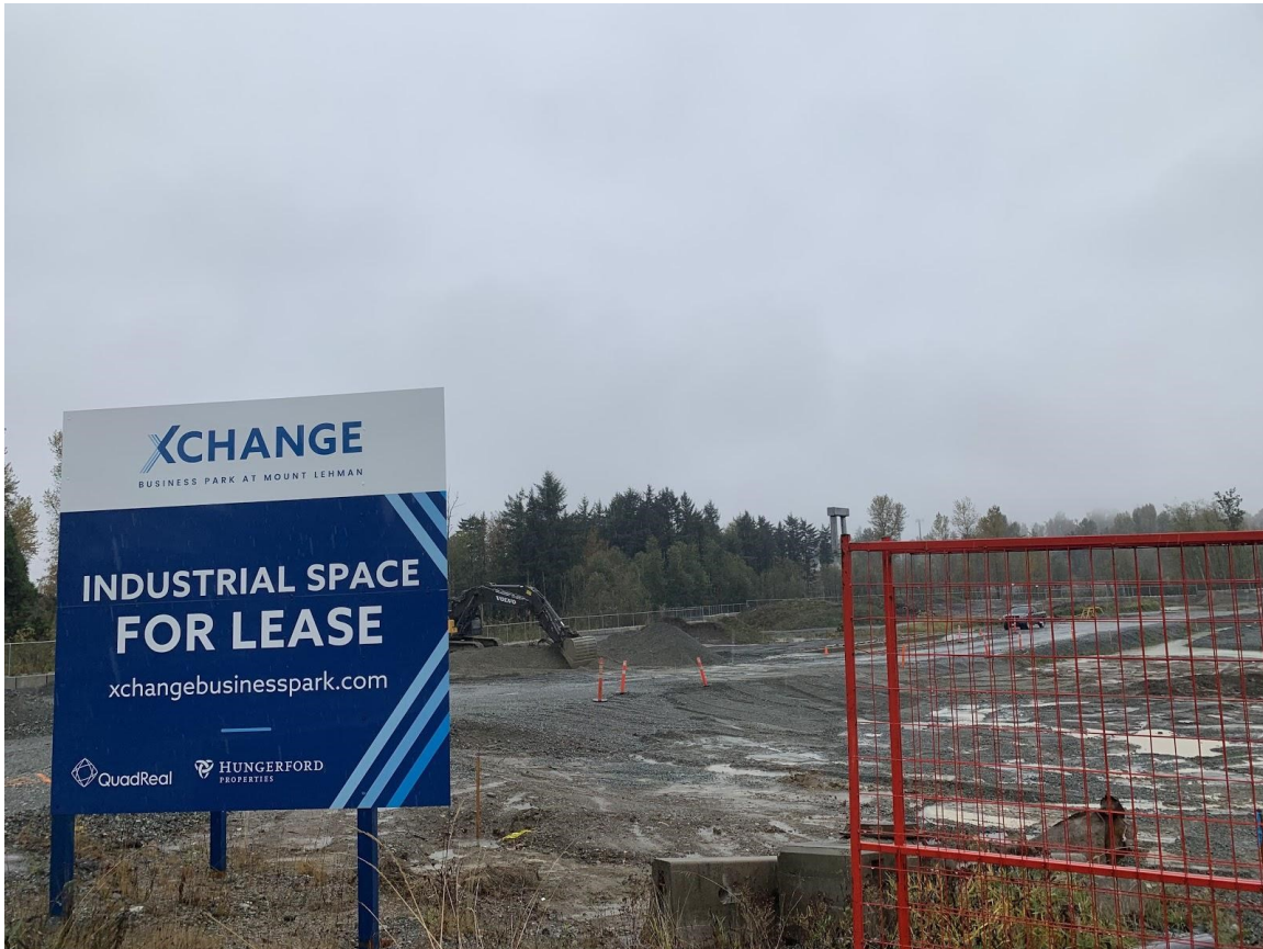
Figure 6-3. Construction of Xchange Business Park in Abbotsford
