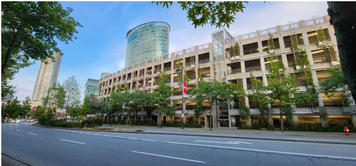
Figure 35. Surrey Central City Parking Structure © Brad Ingram, 2022
