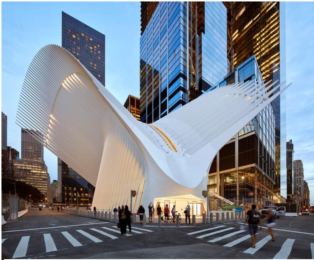
Figure 20. Santiago Calatrava's Oculus at the World Trade Centre. Hufton + Crow, 2017
