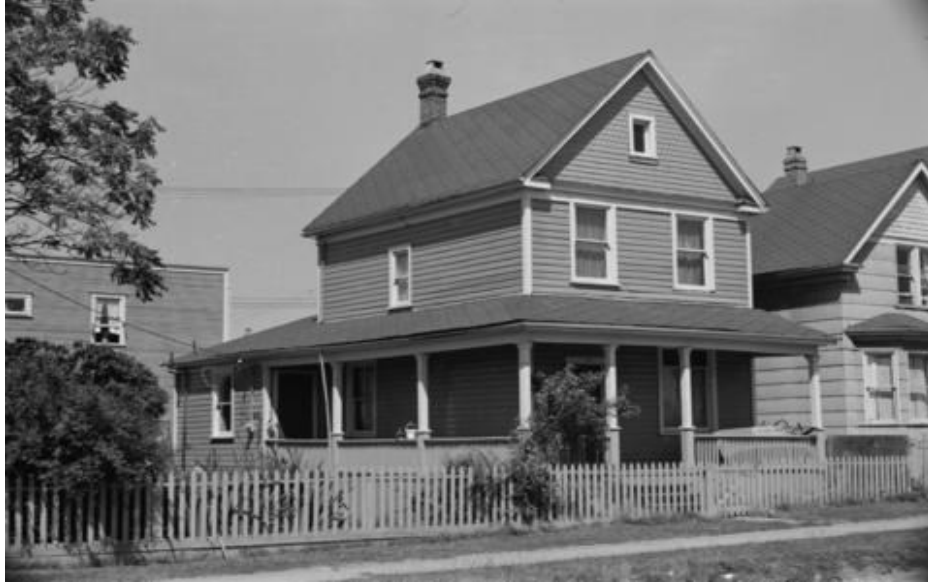
Figure 3.4. 1109 E. Pender Street
