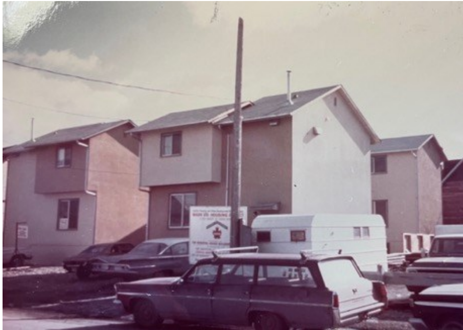
Figure 6.2. Phase II housing
