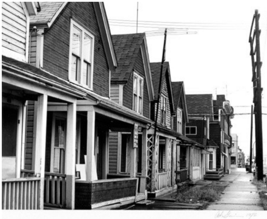
Figure 3.2. 400 block of Heatley Street looking North from Pender Street. Source: These houses were considered too close together and should be demolished. CVA, Art Grise fonds, AM1536-: CVA 70-77 Box 174-D-03.
