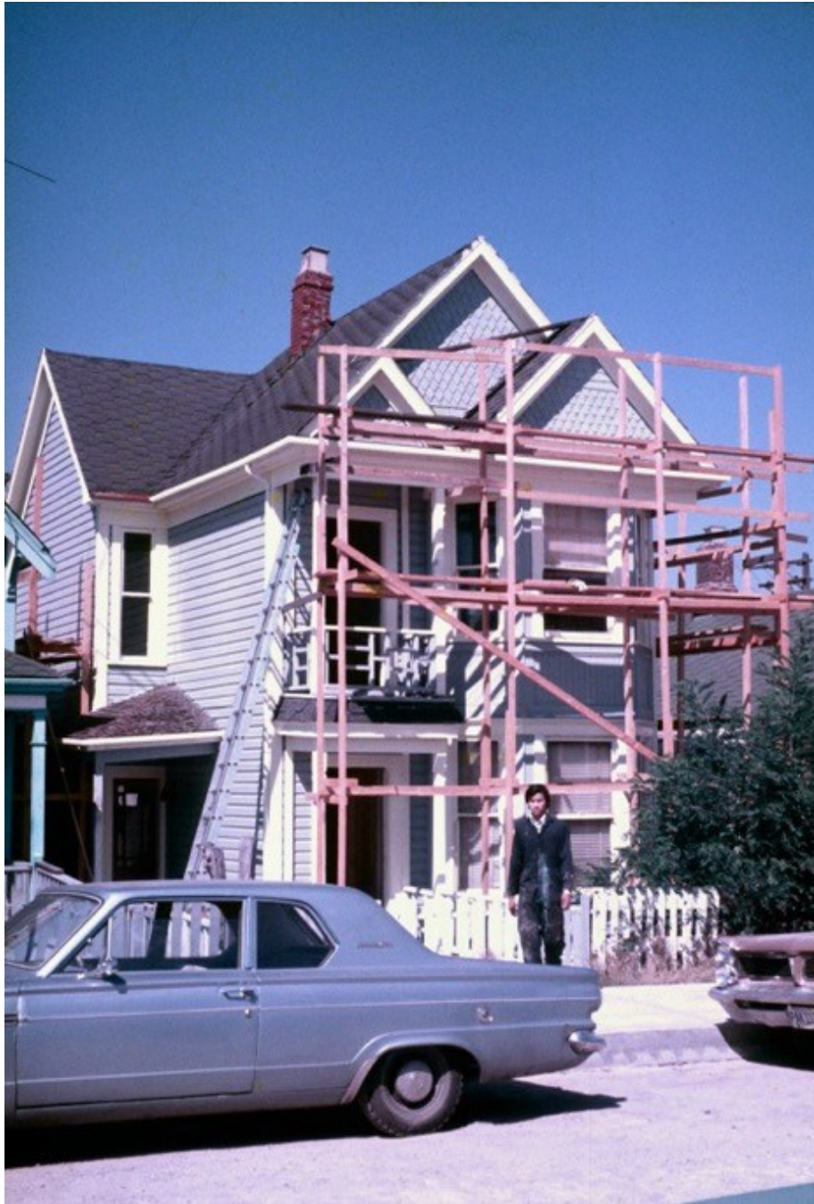
House under renovations in Strathcona, 1973
