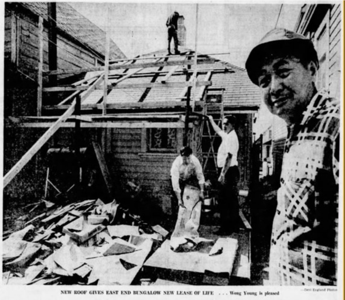
Figure 5.1. Rehabilitation in Action
