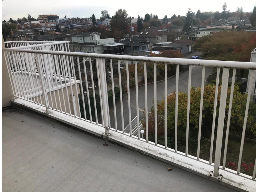
Figure 4.7. 4 th floor communal balcony at LV III
