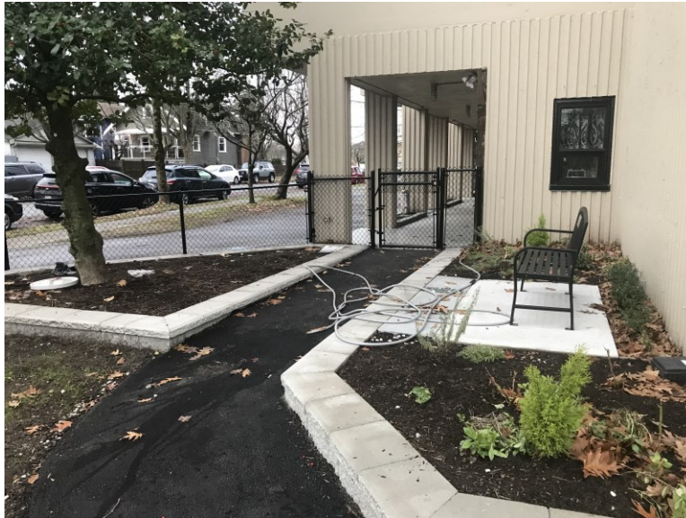
Figure 4.13. Side yard at Collingwood Tower
