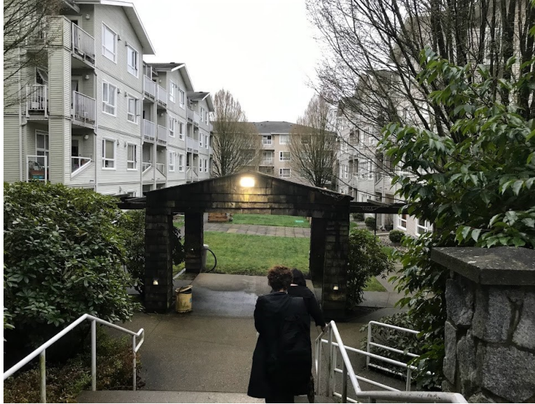
Figure 4.8. Walkways to courtyard at LV buildings
