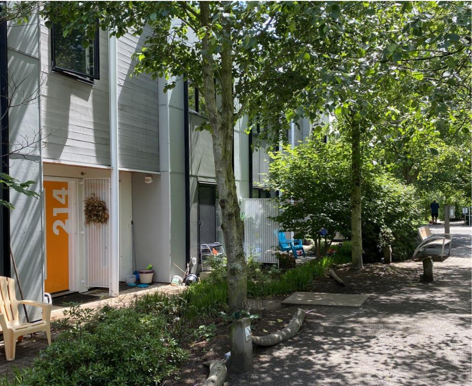
Catalyst's Madrona building, Victoria
