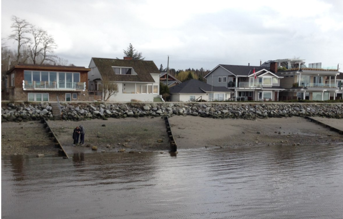
Figure 2: Homes Situated at Elevations Below Dikes and Below FCLs, Crescent Beach (Chang, 2017).
