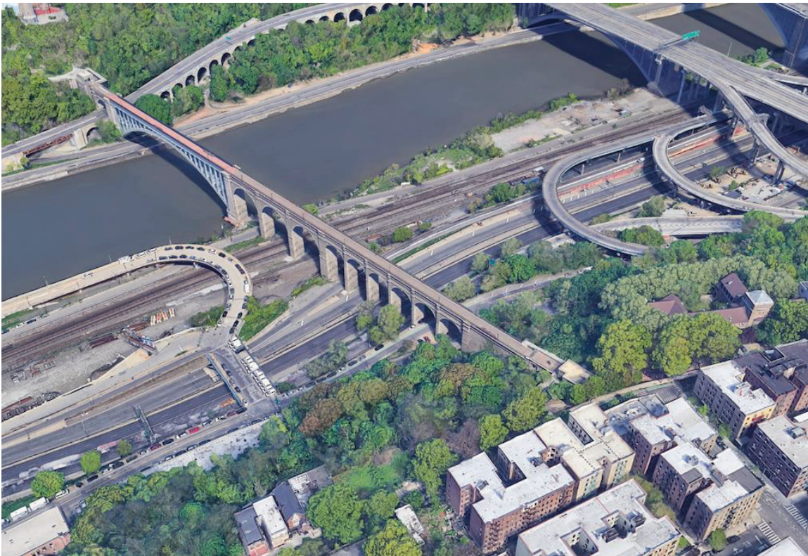
Figure 1.1 Aerial view of the High Bridge (center) connecting Manhattan (top left) with the neighborhood of Highbridge, Bronx (bottom right). The Cross-Bronx Expressway is visible crossing the Harlem River (top right) and the Major Deegan Expressway is visible passing under the High Bridge.
