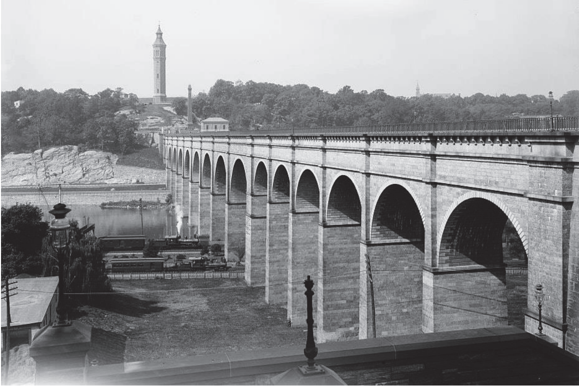
Figure 1.2 The High Bridge in 1900, view West from Highbridge, Bronx to Manhattan. Several stone arches were replaced with a steel arch span in 1928 to allow for large ship navigation of the Harlem River. Source The New York Times .
