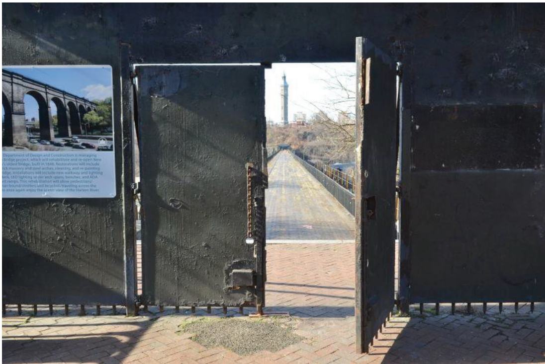
Figure 1.3 View West through fence across the closed High Bridge prior to restoration.
