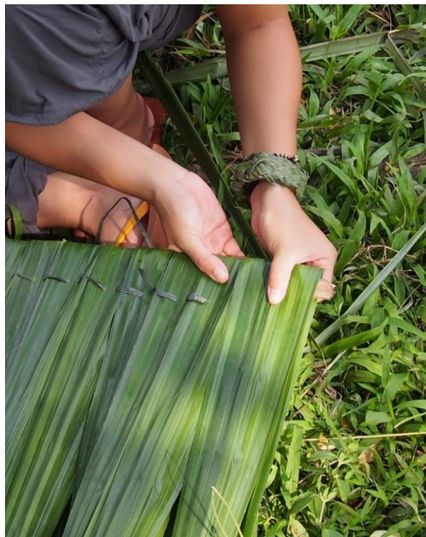
Image 4. Learning to make roofing out of lumbiya leaf w/Kaulo community; Photographed by Tin Gamboa
