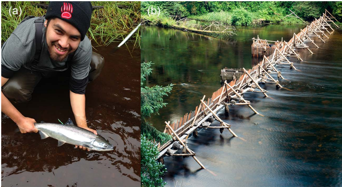
Figure 2.2 (a) Heiltsuk weir technician Richard Wilson-Hall releases a tagged sockeye. (b) The Koeye River weir pictured during June of 2015. The weir is built entirely from locally sourced materials and readily available construction supplies. Courtesy of B. DeRoy.
