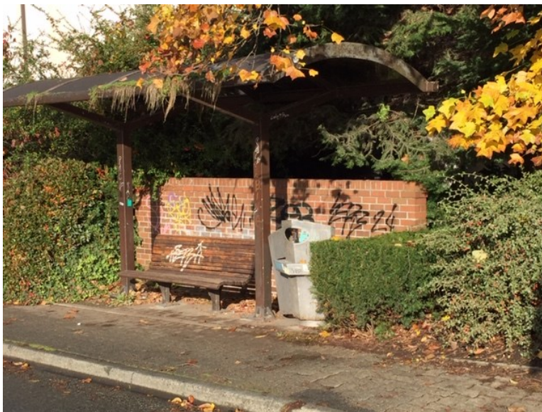
Figure 5.8. Transit infrastructure: Bus stop #50
