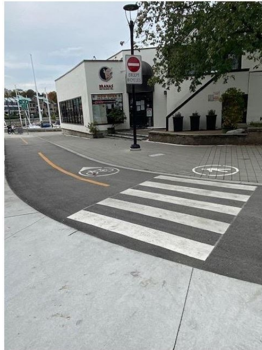
Figure 5.15. Confusing and dangerous intersection on the seawall
