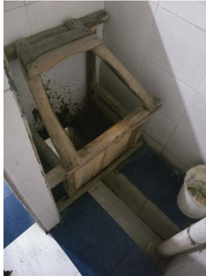
Figure 5 previously existing toilet featuring a frame for elderly to sit upon
