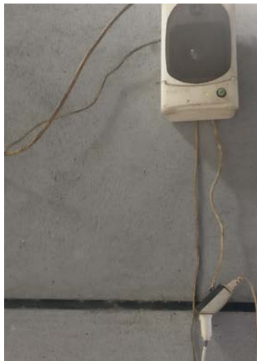
Figure 3 Example of small loudspeaker that is no longer functioning
