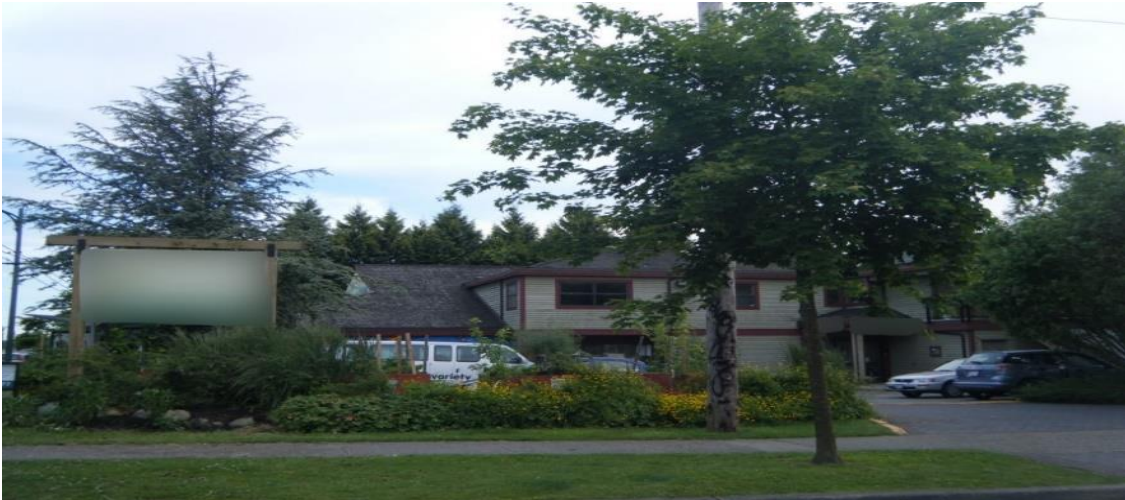
Figure 5.4 Neighbourhood House – entrance
