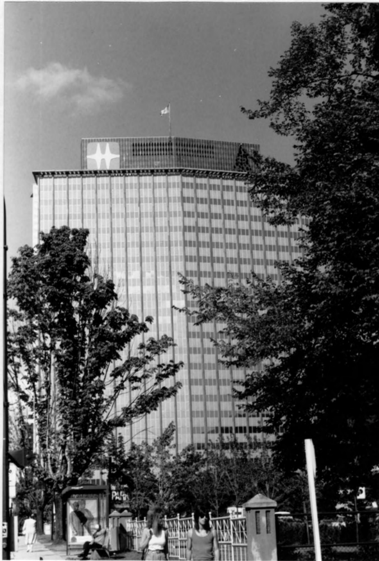
B.C. Electric Company by Thompson, Berwick and Pratt, 1955 – 57.
