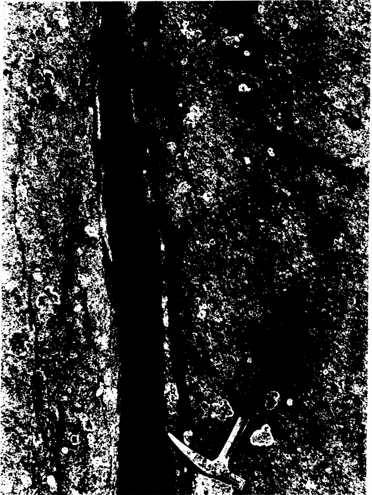
Photograph 26. Induration along an interior joint plane. This has not been previously reported by others studying granitic weathering residuals.
