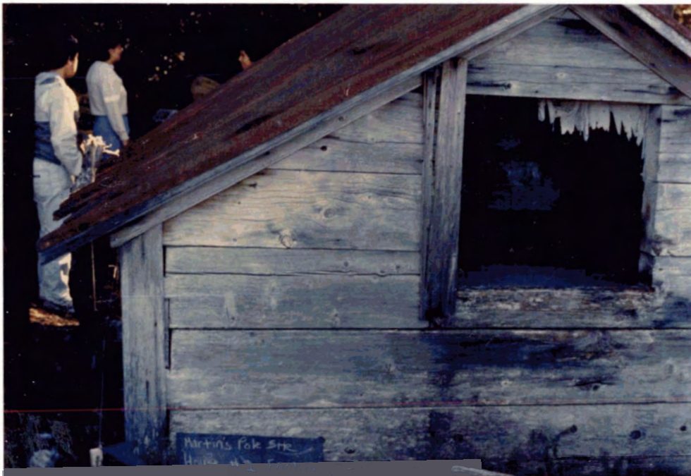
Shirl Hall photos - Features Project - 1985
