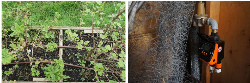
Figure 7.10. The irrigation system for common areas.
